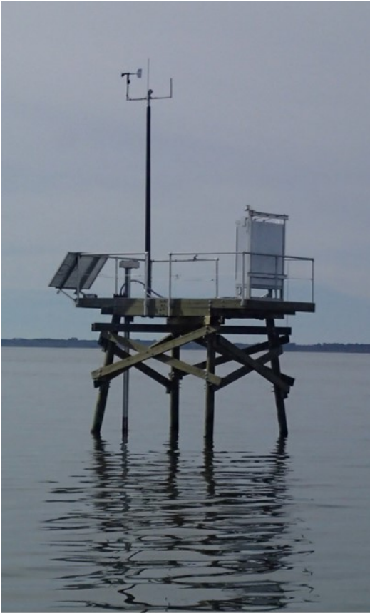
Figure 2: CS05 monitoring platform.
